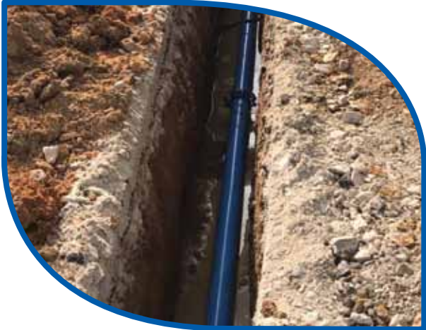
HYPRO® PVC-O for pipe replacement project in Johor
