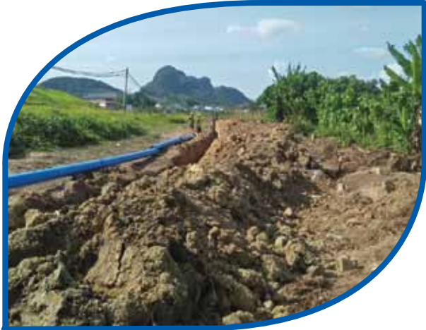
HYPRO® PVC-O for JKR Central Spine Road project in Kelantan
