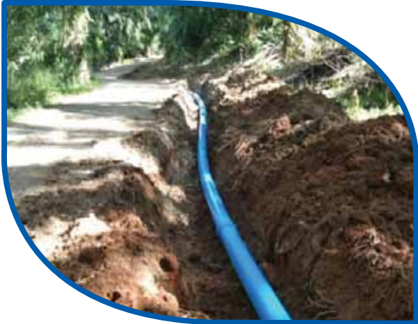
HYPRO® PVC-O for Rural Water Supply Project in Sabah
