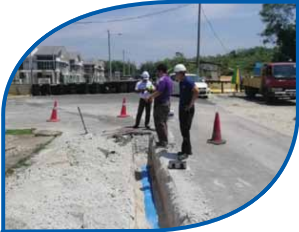
HYPRO® PVC-O pipe for water external reticulation system in a private housing project in Selangor
